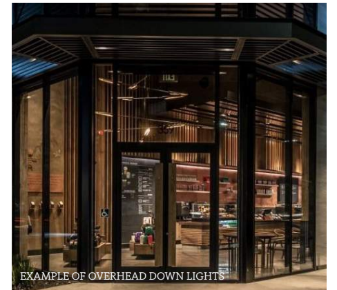
EXAMPLE OF OVERHEAD DOWN LIGHTS & PATH LIGHTS
