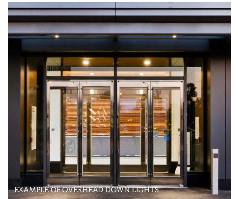
EXAMPLE OF OVERHEAD DOWN LIGHTS
